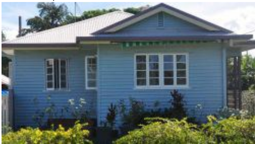
Figure 6.58 - 1950s Post War Expansion precinct (Parsons Street)
